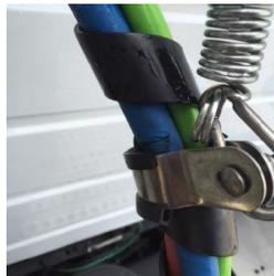
*Field Photo: Clamp Over Tightened to Closed Position*
